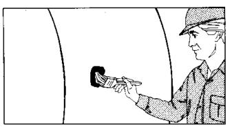
**3.3** Coat all holidays, damaged laminate, and/or exposed steel surfaces using touch-up kit furnished by tank supplier. Follow manufacturer's instructions for mixing and application of resin. (See Section 9 for procedure.) All holidays shall be retested at 10,000 volts.
